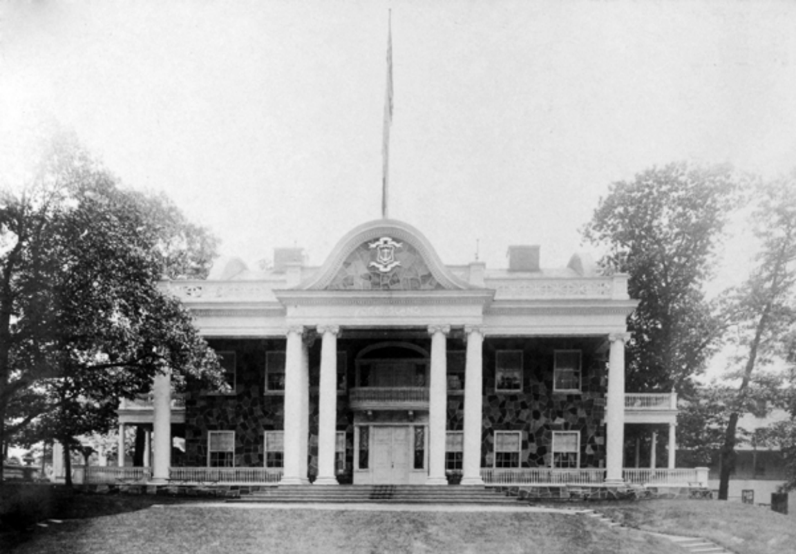
RHODE ISLAND BUILDING
